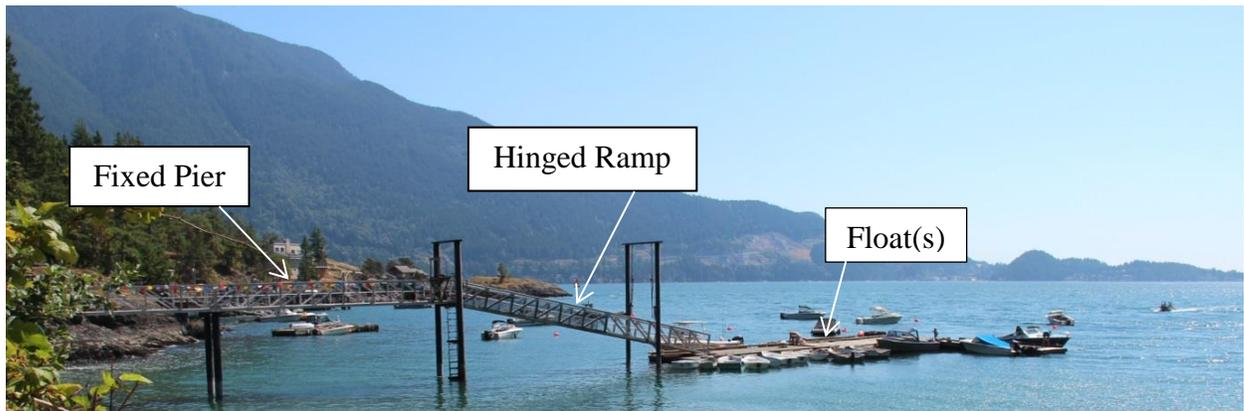
**Figure 1 Typical Three Component Dock Installation on the BC Coast**
